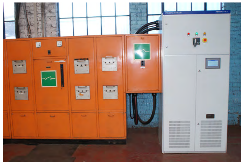
The picture below show the 266kVAr LV STATCOM installed at the VAE SA plant in Isando, Gauteng.
